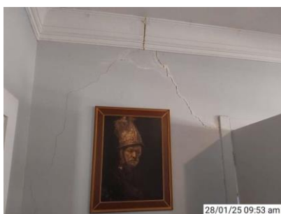
Internal wall cracking
