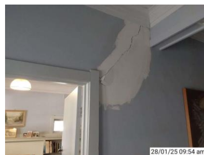
Internal wall cracking
