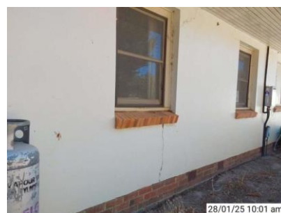
External wall cracking
